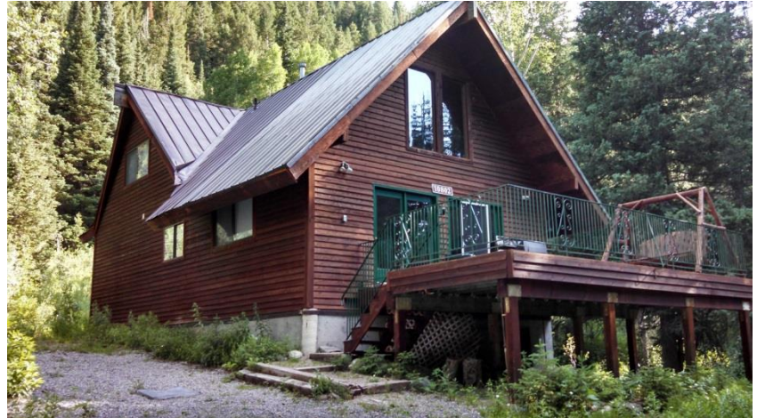
Figure 16 Merrill Maxfield Cabin in Pine Tree Subdivision, Big Cottonwood Canyon on June 27, 2015.
